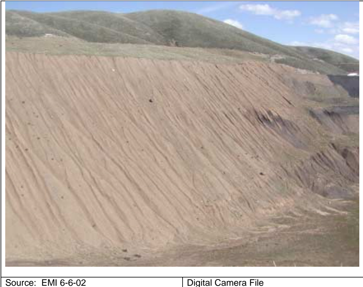
Figure 19-46 Debris Visible in the Eroding Backfill Material of FF / HH Pit
