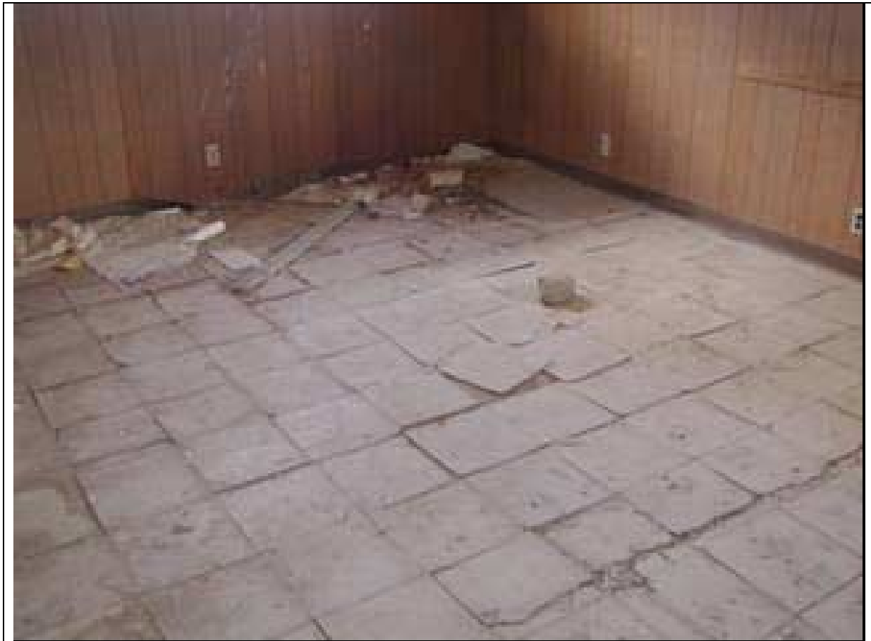
Figure 19-18 Floor tiles in Office Building, Headquarters Area Tiles may contain asbestos
