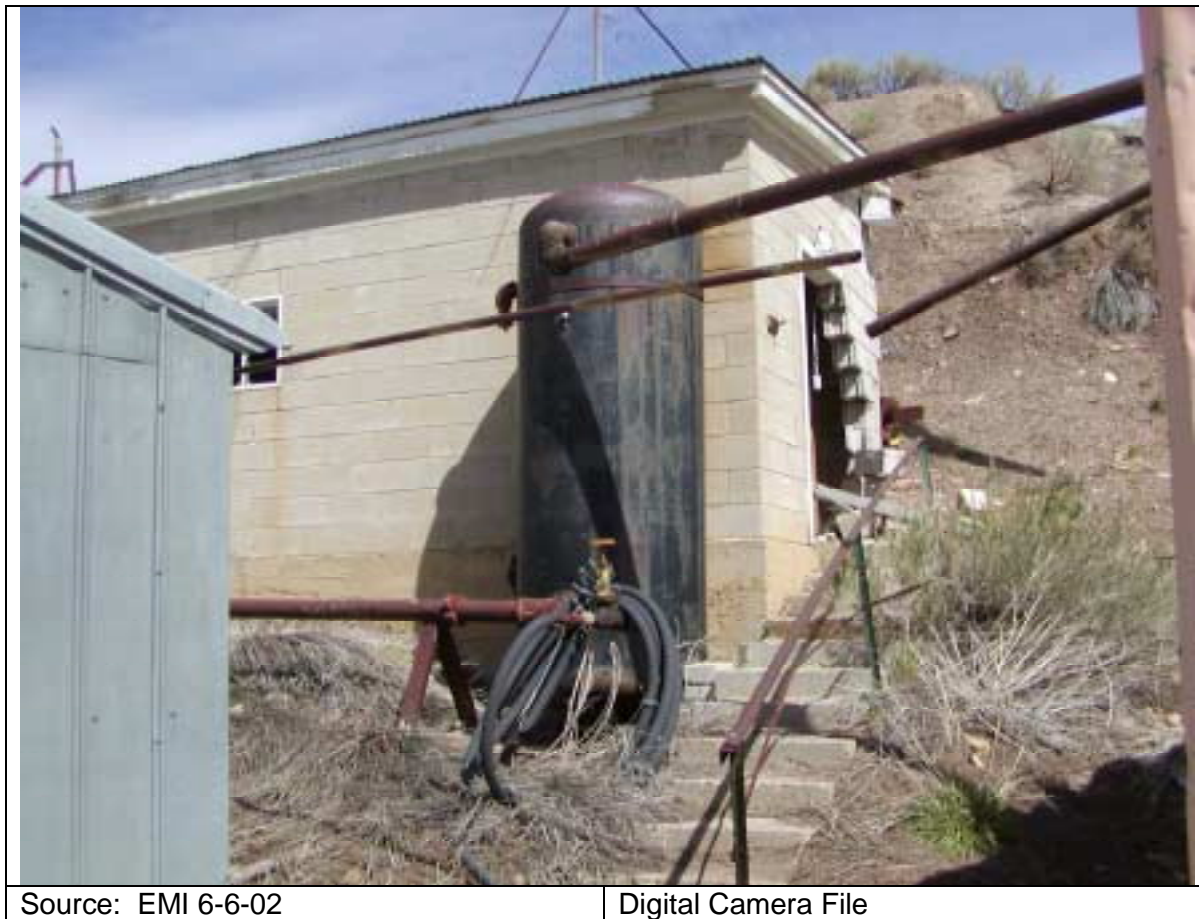
Figure 19-26 Pressure Tank and Piping, Western End of Tipple Petroleum staining was observed on the soil in this area.
