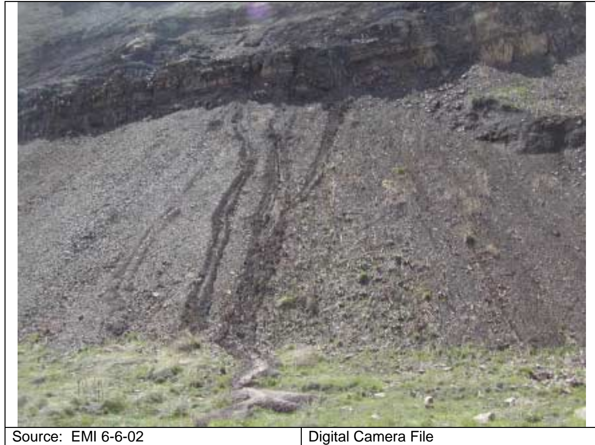
Figure 19-31 Eroded Highwall at C Pit in North Limb View to east. Dark-appearing trails are meltwater flow paths. Note alluvial fan where shale has been deposited by water.
