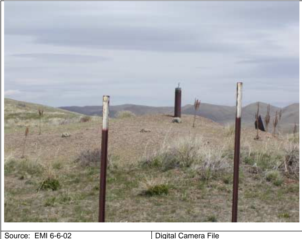
Figure 19-36 Vent Above Explosives Magazine in North Limb
